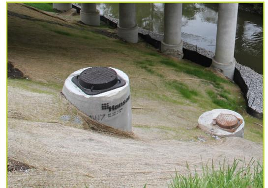
Engineers at MMM used PCSWMM for Stormceptor to properly select and size each Stormceptor unit, based on the site's five drainage areas and pollutant removal requirement. PCSWMM for Stormceptor provides a detailed technical output that can be submitted with an MOECC ECA application, with unit technical specifications and drawings available online. Re-sizing can also be easily undertaken if a site's drainage parameters change, which is common during the life of a major project.
